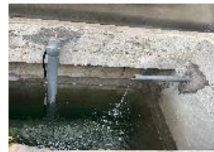
Water from water dispensers, air compressors, rainwater, and glass cleaning machines converge into a 50-ton water tank.
